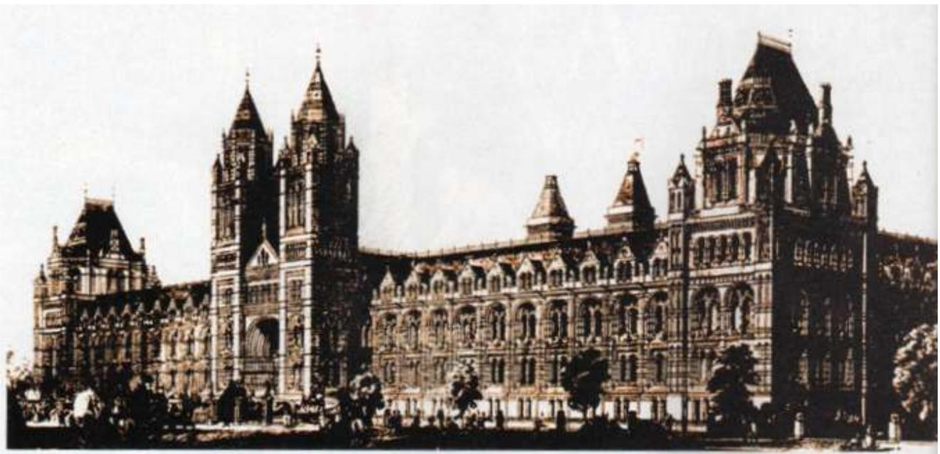
Figure 3: The Natural History Museum in London England completed in 1881 relied on six towers to passively ventilate the building. The four front towers are shown in this graphic. Reprinted with permission from the ASHRAE Journal.
